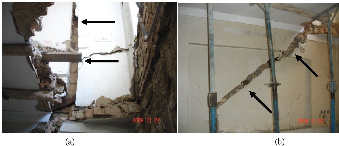
Figure 2: Sample of crack paths and point classification.
