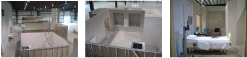
FIG 1. Mock-ups of selected hospital rooms ( http://www.arnett.com/camc.html ).
