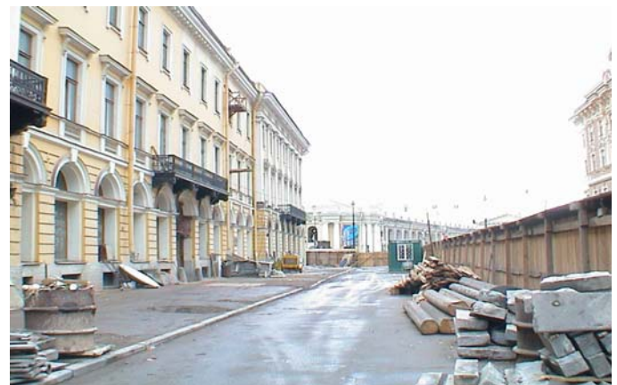
Figure 7. Promstroibank St Petersburg, Russia - north façade
