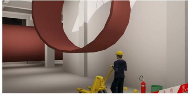
(b) Ice-storage Cooling Tank Installation Simulation
