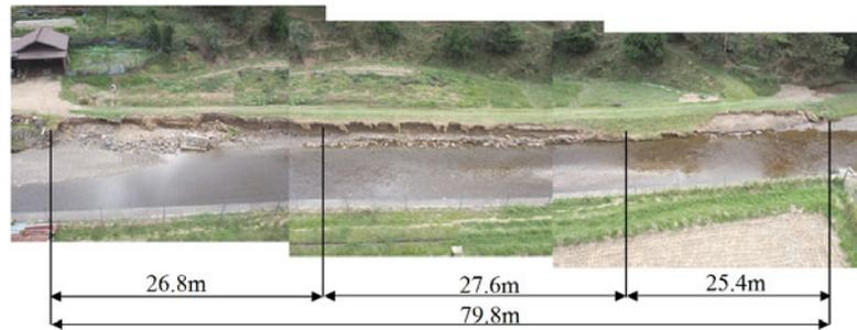
**Figure 10. The damaged river bank in Kyoto Prefecture**
