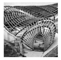
Fig 4. Use of ruled surfaces in the Water Pavilion by NOX.
