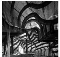
Fig 2. Structural frames in Gehry's building in Seattle produced by contouring.
