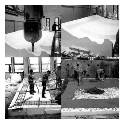
Fig 5. Milling of molds for concrete casting in Gehry's building in Dusseldorf.
