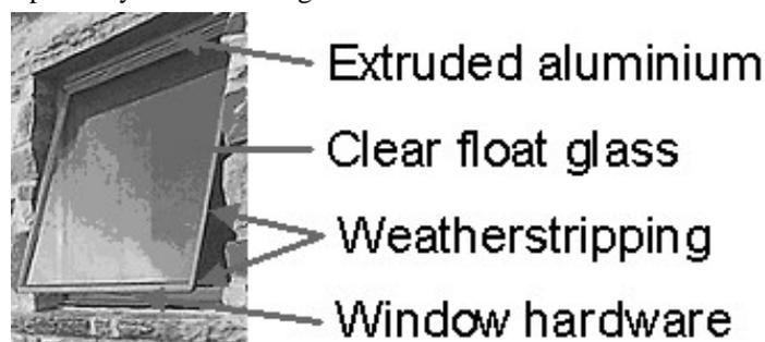
**Figure 1: Components of an Aluminium Window**
