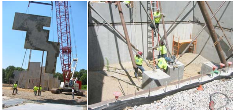
Figure 5: Bracing the concrete panels
