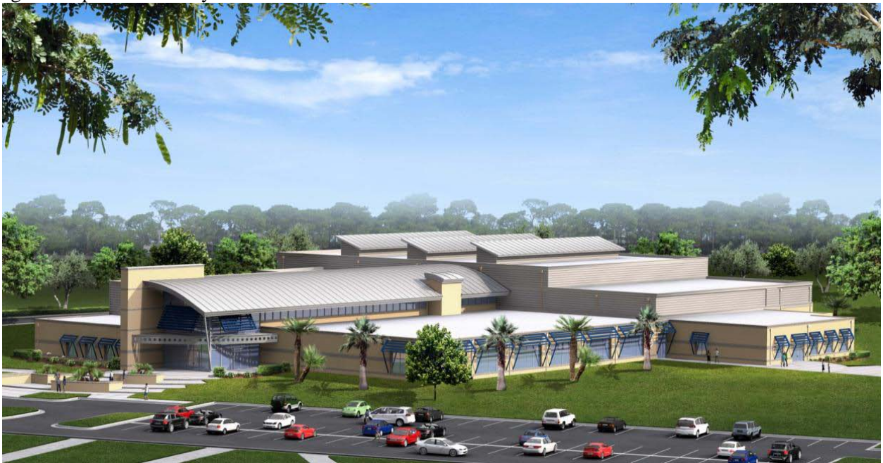
Figure 4: Tyndall Fitness Center, LEED Platinum and BIM-testbed
