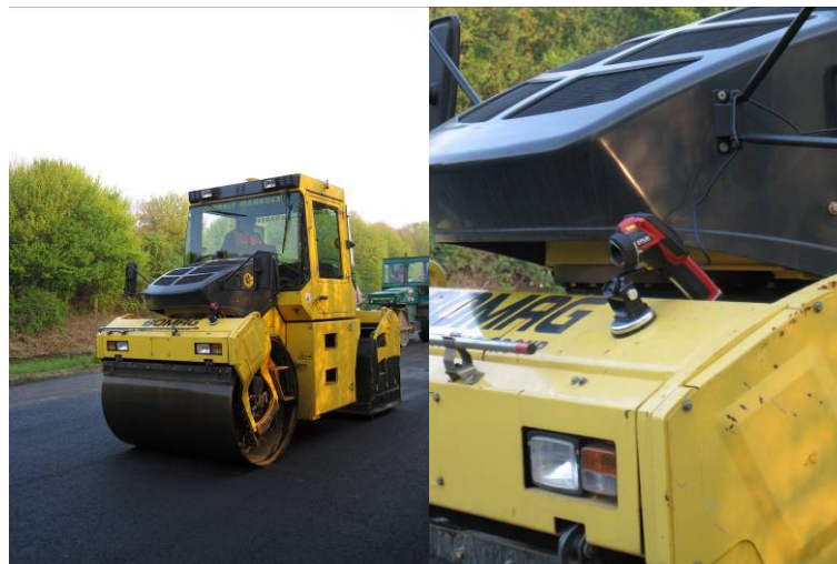
Figure 3: IR camera attached to a roller using magnet
