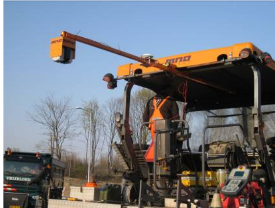
Figure 2: Linescanner mounted behind a paver
