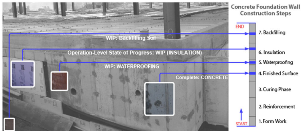
Figure 1. Example of operational-details for constructing a concrete foundation wall and how monitoring can benefit from detecting appearance information.
