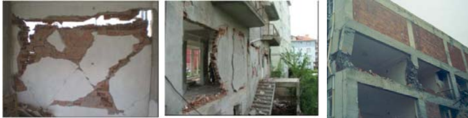
Figure 3. Typical out-of-plane failure of URM infills in RC framed building, showing top-down collapse creating new voids that reveal the underside of the RC beams.
