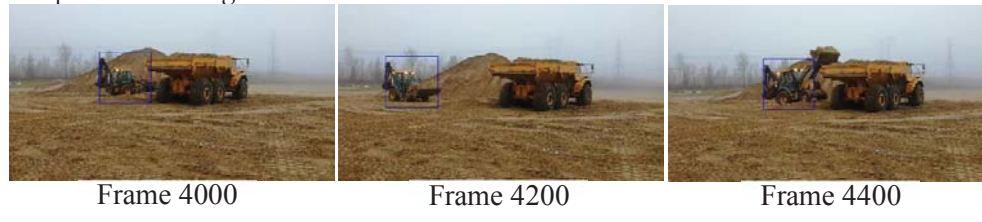
Figure 6: Tracking results of the backhoe
