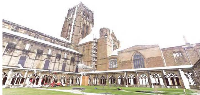
Figure 2: Example of captured laser scan data of Durham Cathedral
