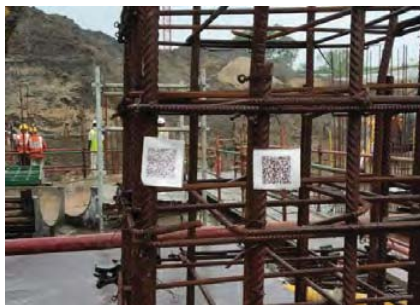
a. QR codes fixed on the rebars
